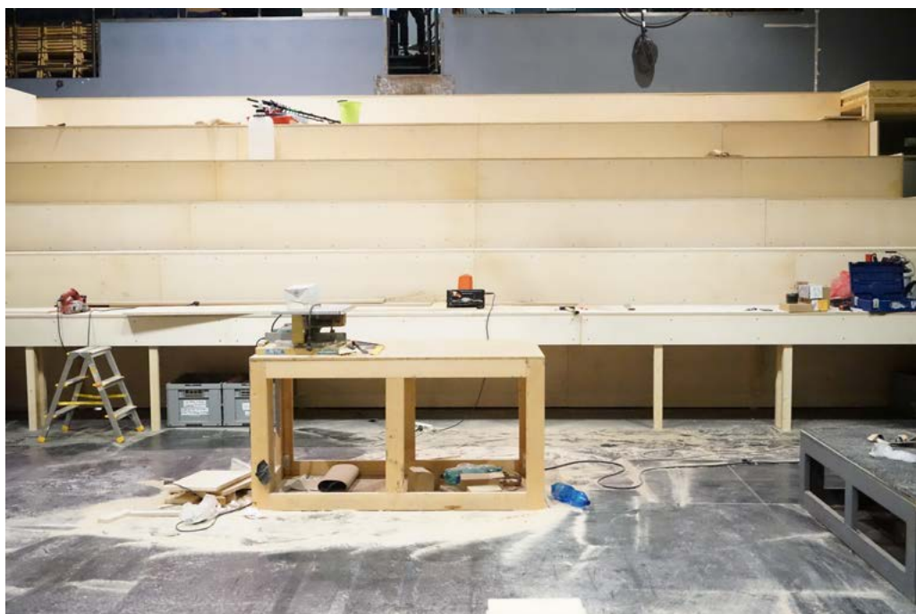
Stavba nové elevace / Construction of the new seatings
